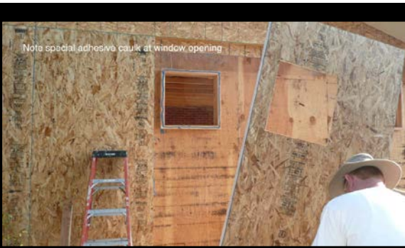
Figure 7. Retrofit Panel Routed for Window Box
