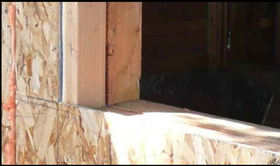
Figure 7. Retrofit Panel Routed for Window Box
